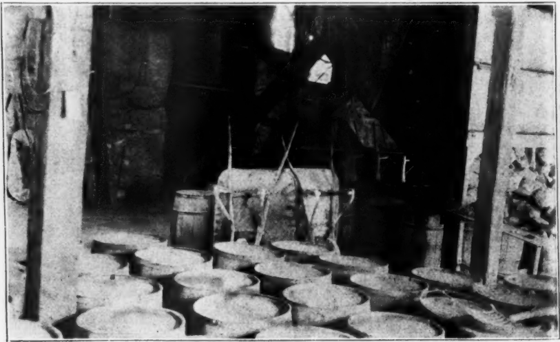
Incline From Bottom of Kiln Showing Storage Tank
